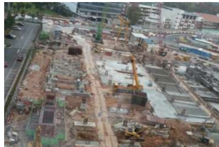
Ground slab construction in-progress
