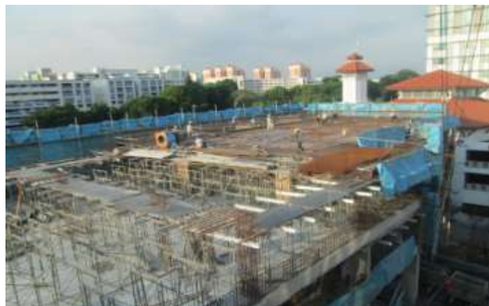
▲ Formwork and rebar installation
