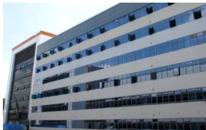
▲ New 6-storey extension wing
