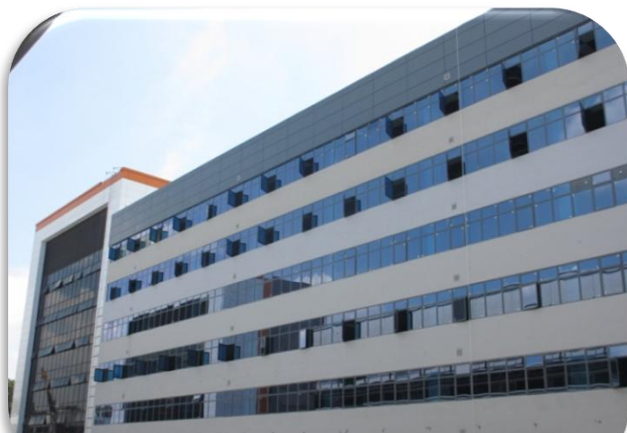
Completed 6-storey extension wing
