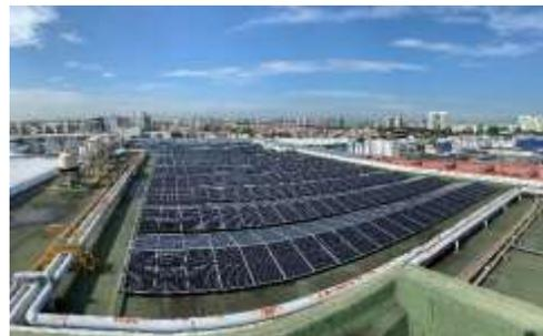
*The total generating capacity of solar panels at Serangoon North Cluster and K&S Corporate Headquarters is 848.8 kWp.*
