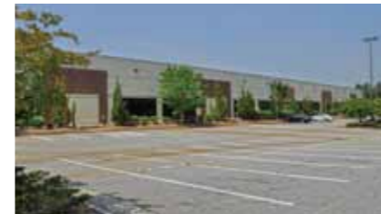
51 1805 Center Park Drive Charlotte, North Carolina
