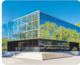
3 2601 West Broadway Road, Tempe
