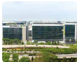
66 Mapletree Hi-Tech Park @ Kallang Way
