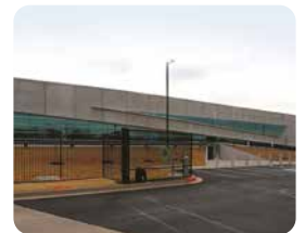
35 4121 & 4114 Perimeter Center Place, Oklahoma City
