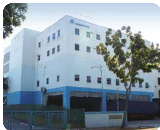
97 2A Changi North Street 2
