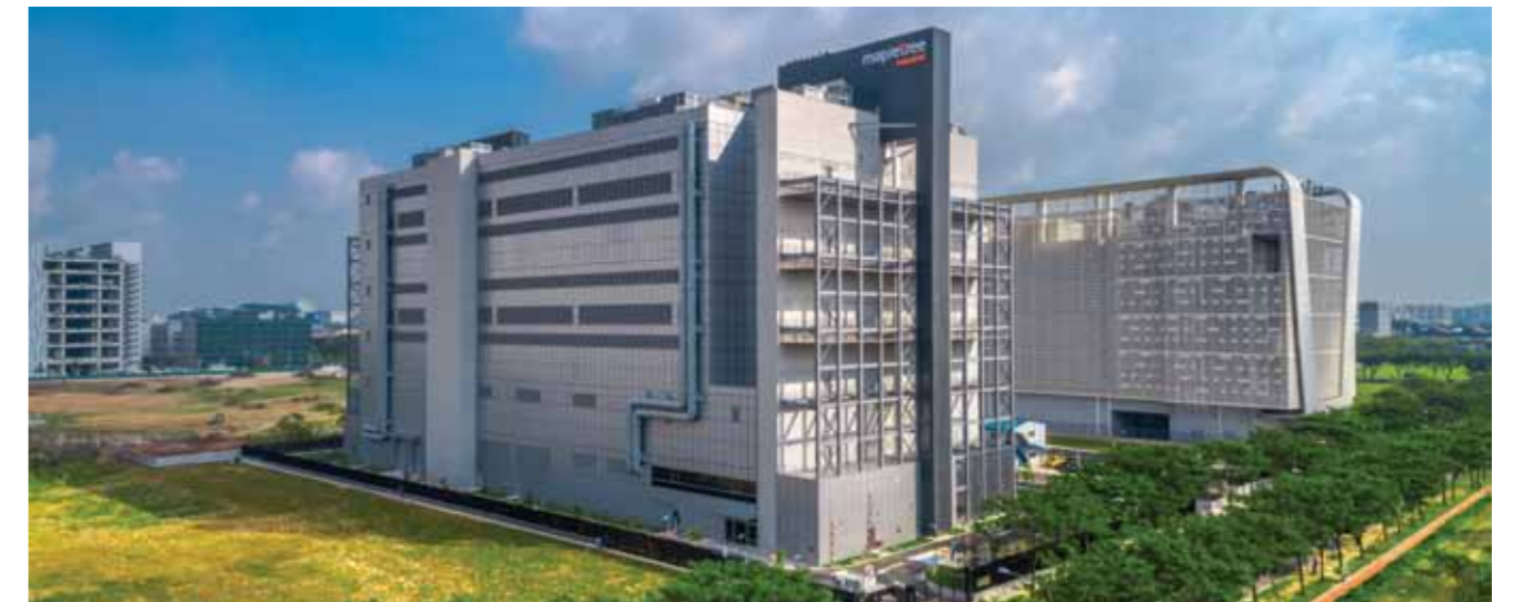
Third BTS data centre development, Mapletree Sunview 1
