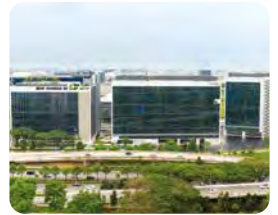
66 Mapletree Hi-Tech Park @ Kallang Way
