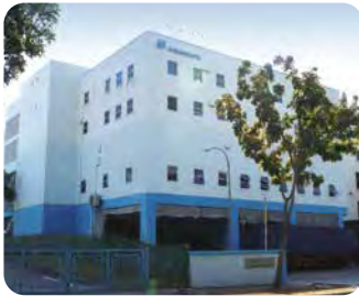
97 2A Changi North Street 2
