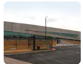
35 4121 & 4114 Perimeter Center Place, Oklahoma City
