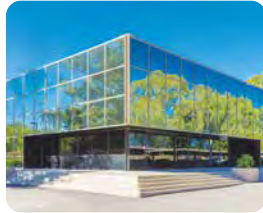
3 2601 West Broadway Road, Tempe
