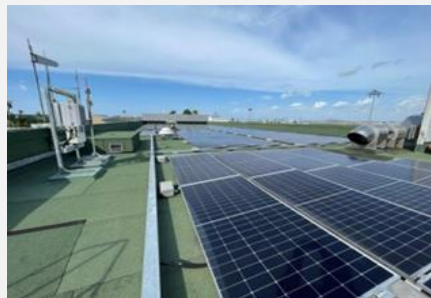
Solar panel installation at 50 Airport Boulevard, Singapore
