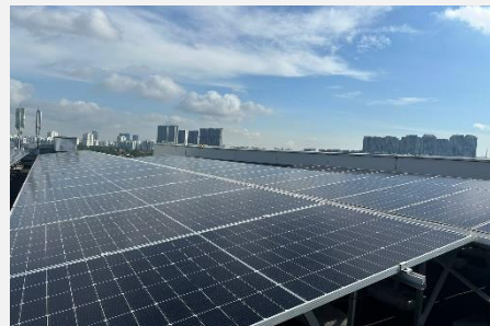
Solar panel installation at 4 Tuas Avenue 5, Singapore
