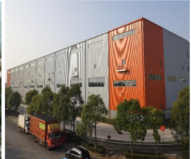
Ouluo Logistics Centre, Phase 1
