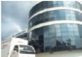
KLW Industrial Building
