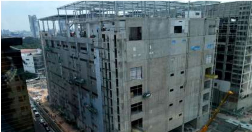
Façade and external works in progress
